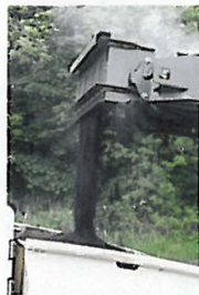
↓ Milled material is deposited into the paver
